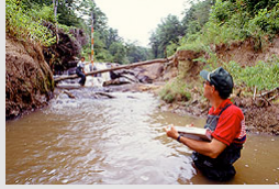
Overflow of embankment
